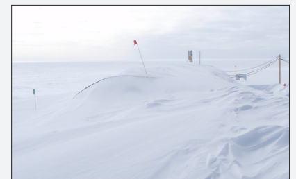
First view of the arch facility by the camp put-in crew. To get a feel for the amount of drifting, this photo is taken looking at the end of the drilling arch, which is 27 feet tall. Photo Credit: Raytheon Polar Services
